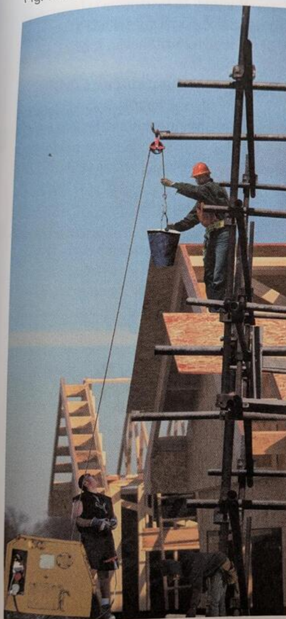
Fig. 1.95 Using a fixed pulley
